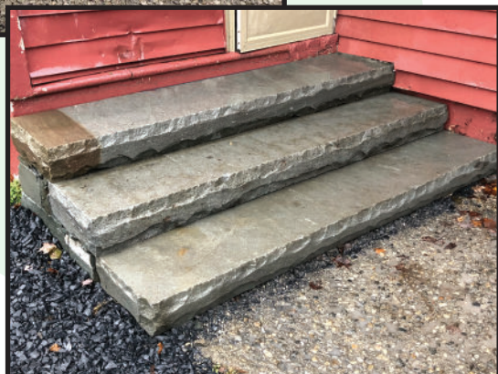
After - 6" Bluestone Steps. Beautiful, and far more durable than concrete.
